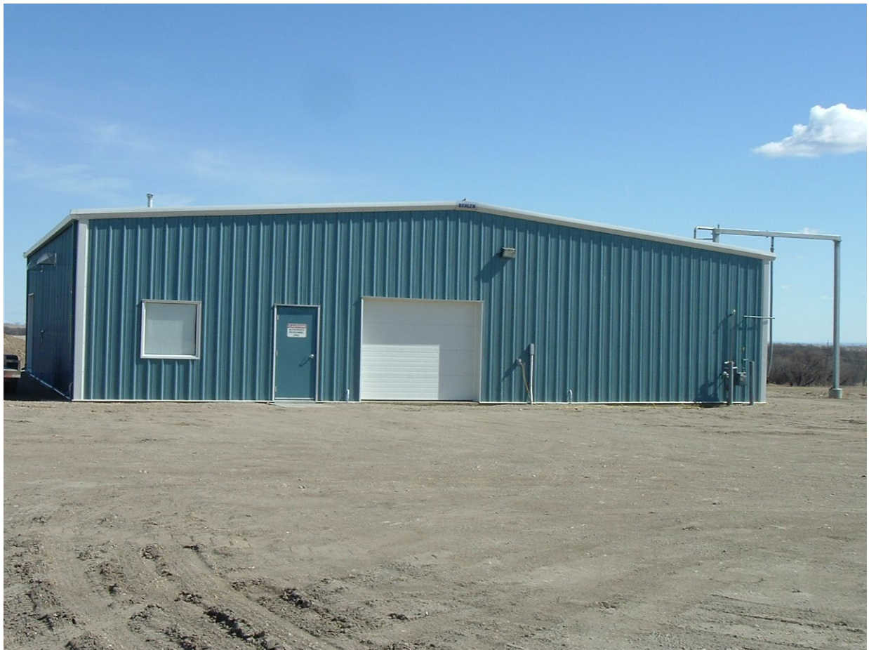
The Melita Water Treatment Plant
